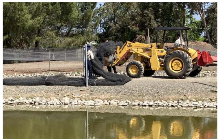
The left picture depicts installing a new solar aerator and the right is setting out a new predatory exclusion net over a fish rearing pond.
