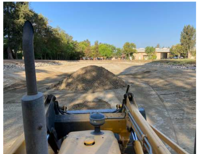
The pictures provided are the process of removing debris from the pond bottom. The sediment and debris are scraped away with the tractor then hauled away with the dump truck.
