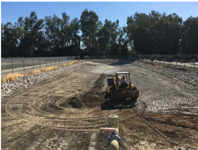
The pictures provided are the process of removing debris from the pond bottom. The sediment and debris are scraped away with the tractor then hauled away with the dump truck.
