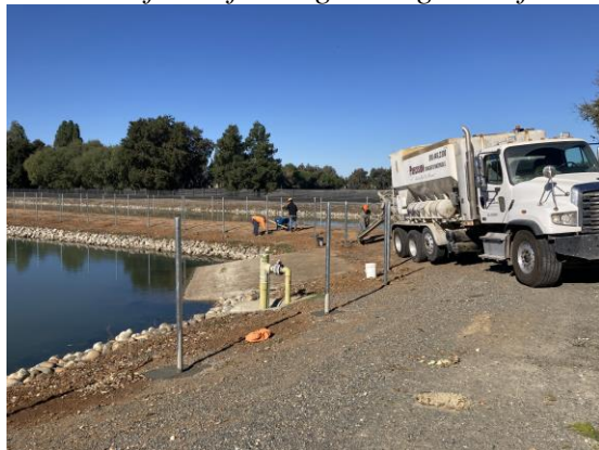
Pictures of new fencing during and after installation.
