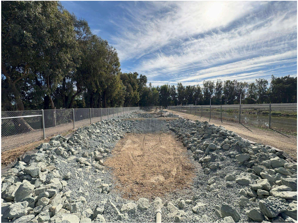
Above: Perch pond lined with riprap and gravel.
