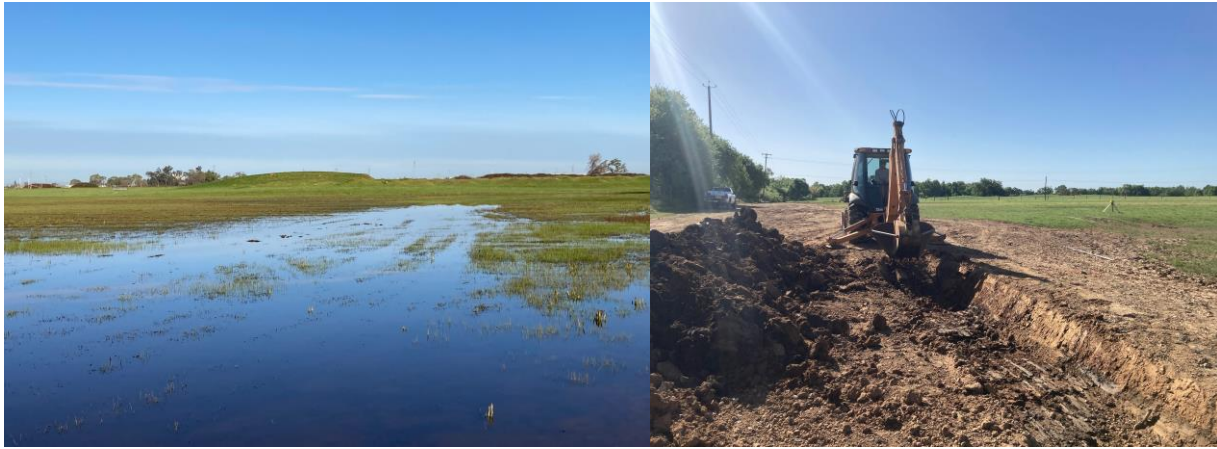
*BMP Project: Pasture drainage ditch being excavated in south Elk Grove
