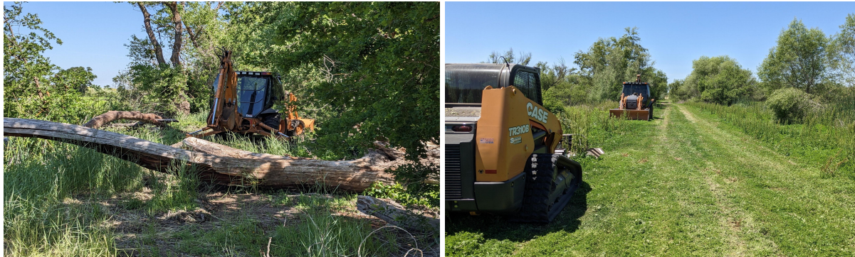
Water Management and Vegetation Management Project: Stone Lakes National Wildlife Refuge
