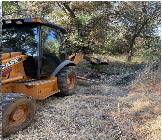
Image: Backhoe removing emergent vegetation
