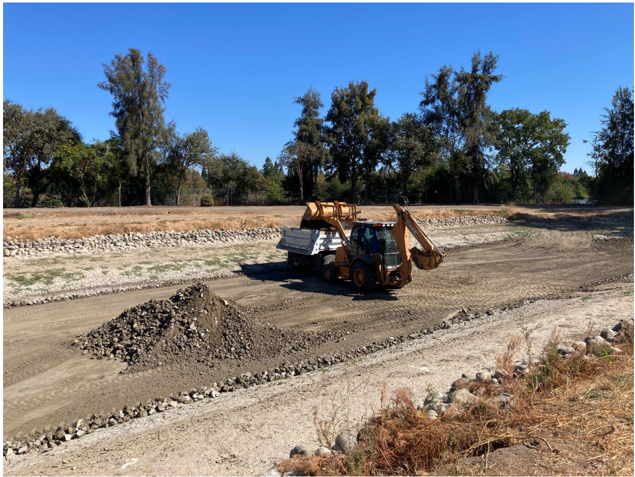
Above : Picture of pond sediment being removed.
