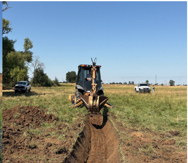
Image: Excavation of new drainage ditch
