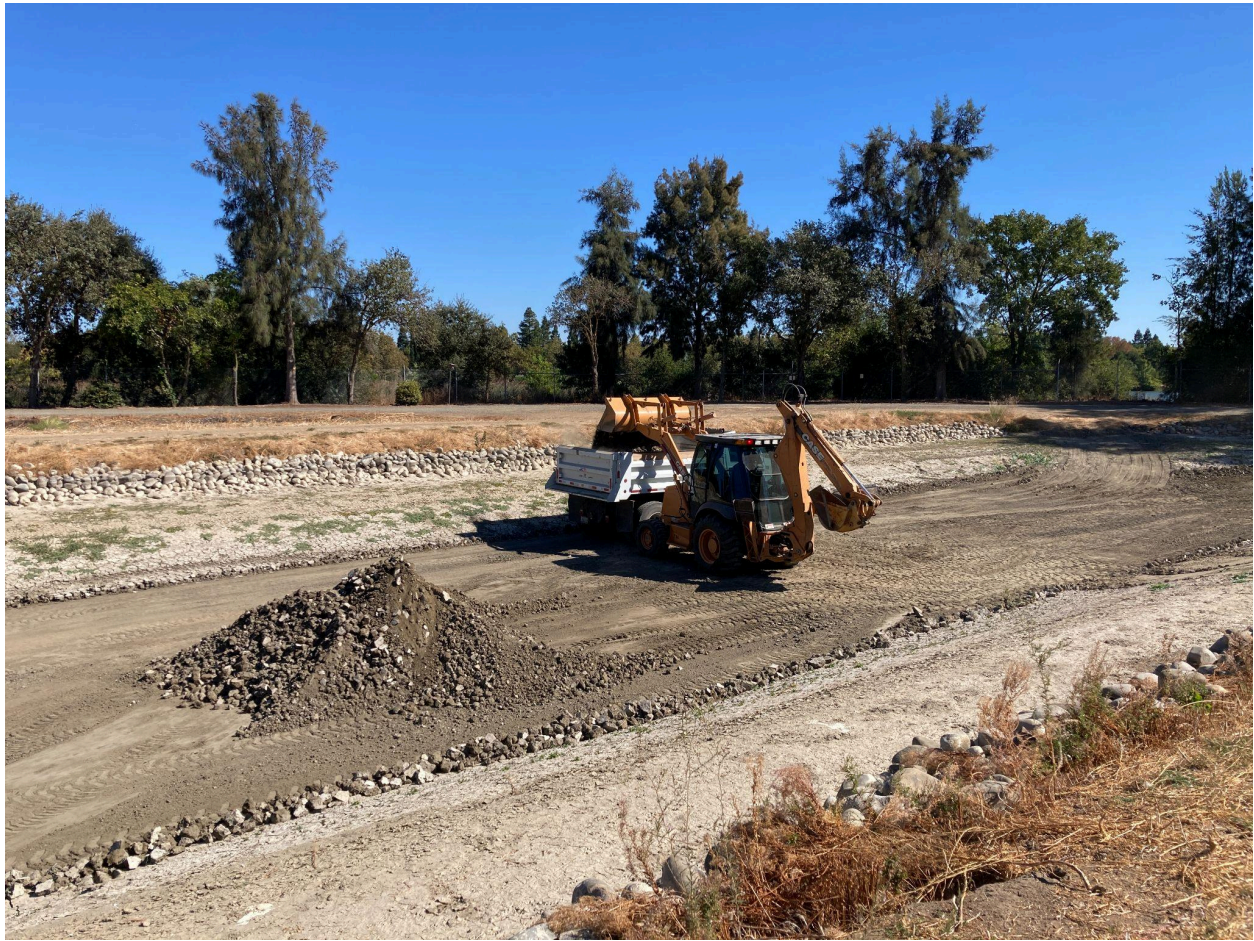
Above : Picture of pond sediment being removed.
