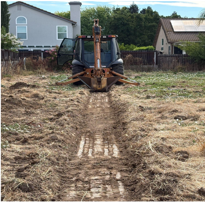
Image: Excavation in progress
