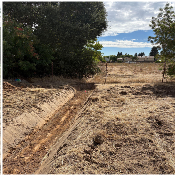
Image: Finished V-ditch
