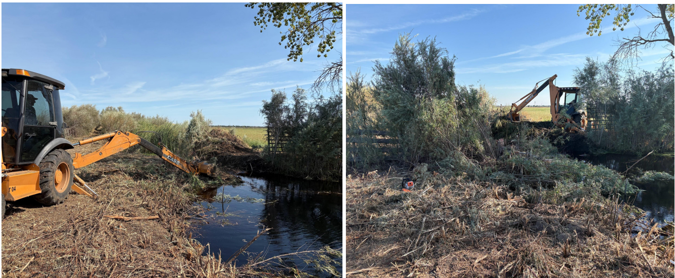
Images: District staff removing beavers dam spoils
