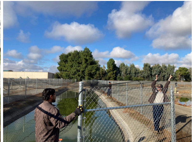
Bottom Right: Picture of a technician's adding netting to cement pond.
