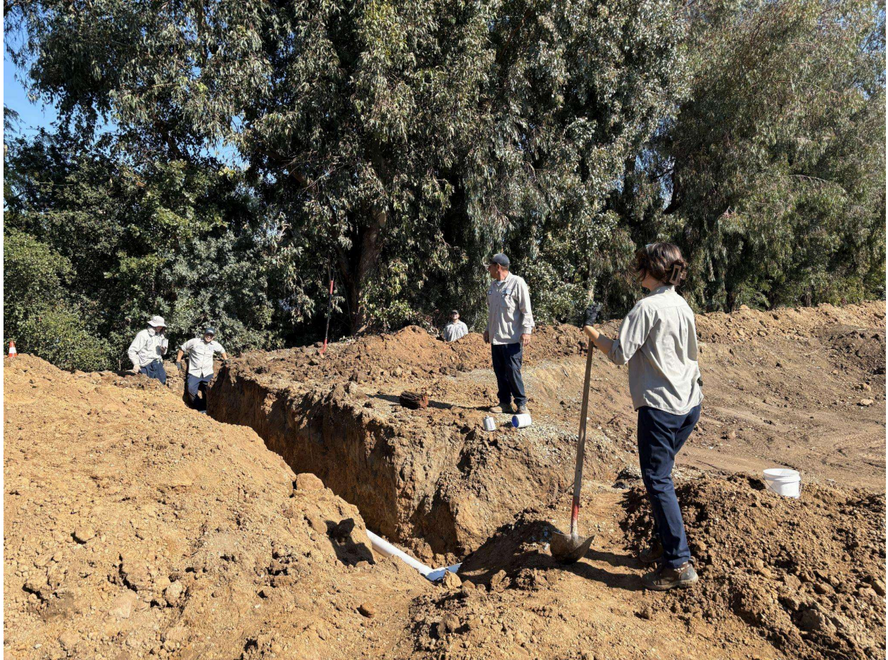
Top and Bottom: Ecological Management and Fisheries technicians installing water lines for the new perch ponds.
