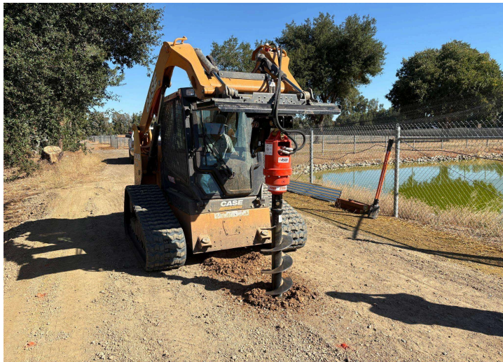
Image: Post hole excavation
