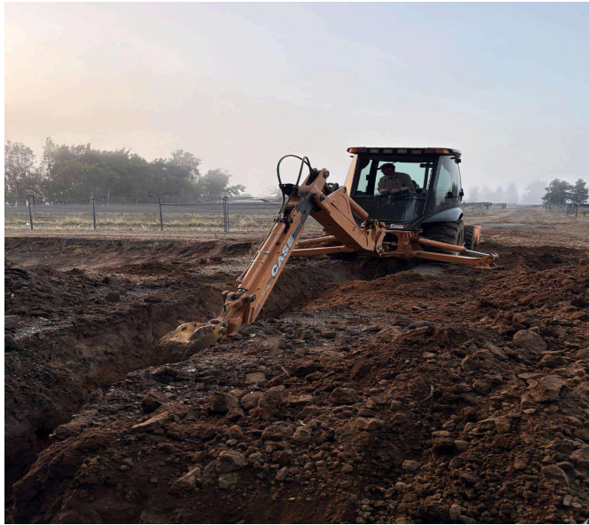
Image: Plumbing Excavation
