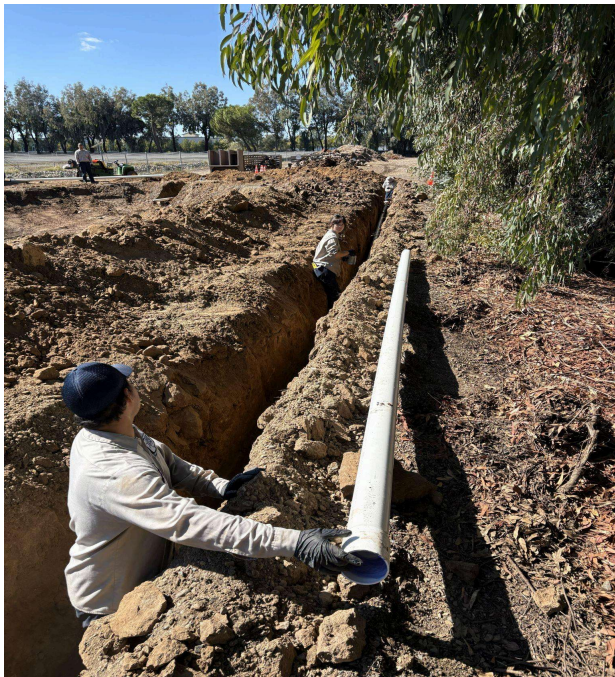
Top and Bottom: Ecological Management and Fisheries technicians installing water lines for the new perch ponds.
