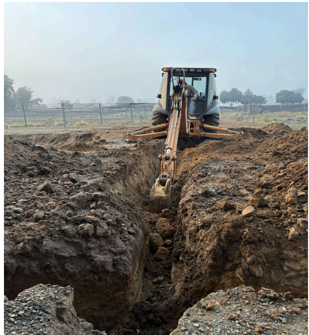
Top and Bottom: Ecological Management and Fisheries technicians installing water lines for the new perch ponds.
