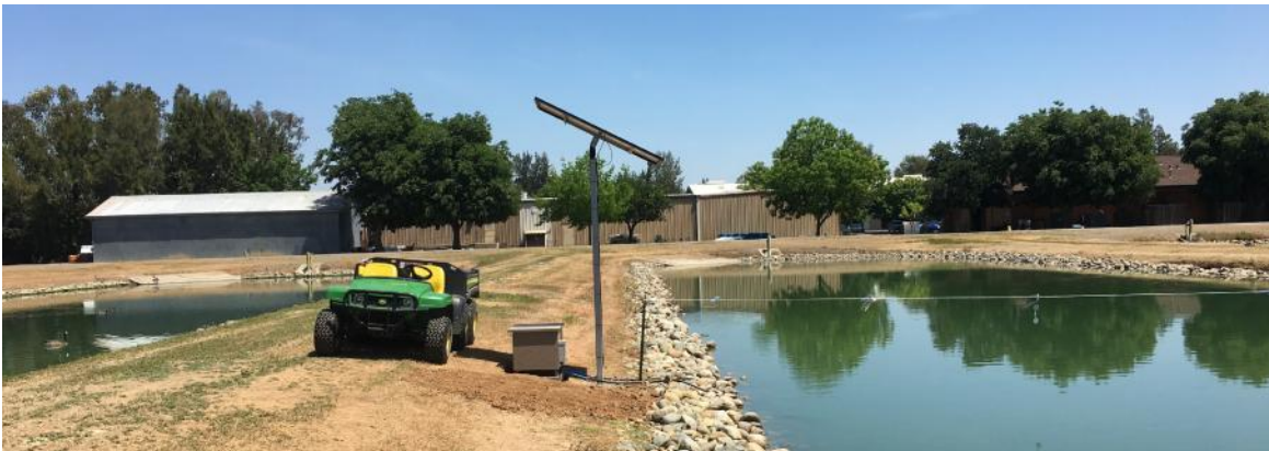
Picture above shows our new solar pond aerator. This aerator is designed to run dusk to dawn when photosynthesis is nonexistent and dissolved oxygen is at its lowest levels. This system will then recharge during daylight hours.
