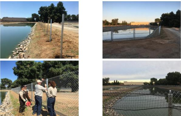
Pond fencing construction: Clockwise: poles placed, fence built, cables installed and lastly predator exclusion net put into place. This new predator exclusion will be monitored here forward for fish yield increase and fish quality.
